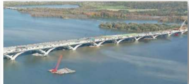
Woodrow Wilson Bridge
